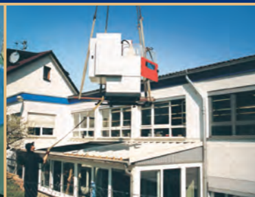
A new CNC wire-cut EDM machine is lifted in over the roof
